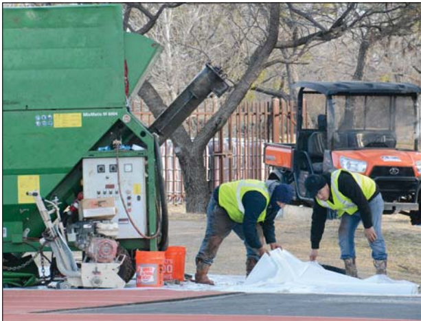
Two construction workers lay down tarps to prepare the track for resurfacing. The track is expected to be completed on Feb. 26. PHOTO BY PARKER MOON
